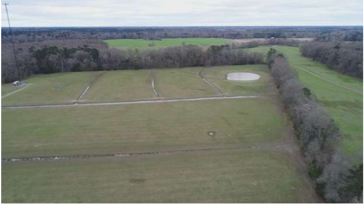
Aerial view (looking east) of southern most portion of the property to be restored; artificial drainage ditch and southernmost stock pond (southeast corner of property) to fill are visible near southeast corner; Proposed Beaver Creek Mitigation Bank (photo taken February 15, 2017).
