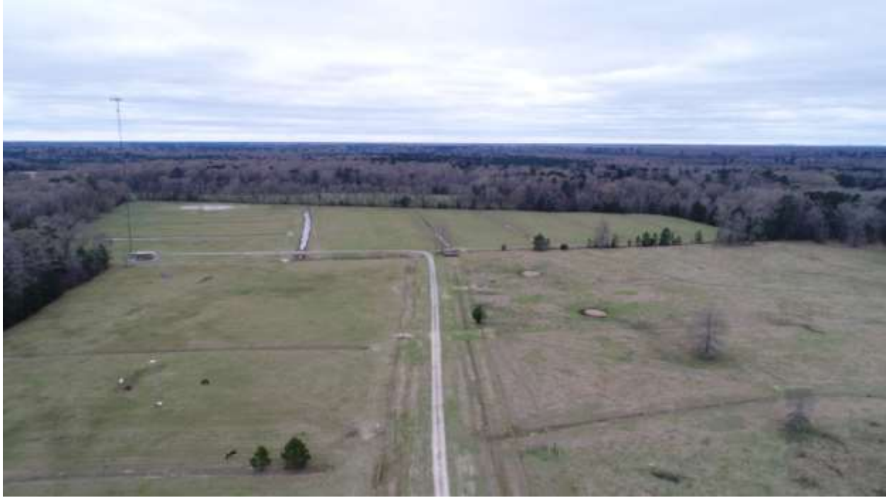
Aerial view (looking south) of drainage alterations in re-establishment/rehabilitation areas and access road/telecommunication facility/tower to remain, Proposed Beaver Creek Mitigation Bank (photo taken February 15, 2017).
