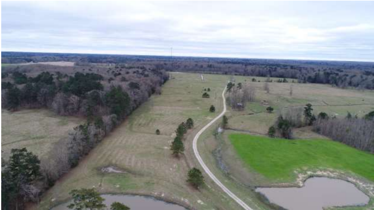
Aerial view (looking south) along access road to telecommunication facility/tower; northern most stock pond to fill on rights side of road; Proposed Beaver Creek Mitigation Bank (photo taken February 15, 2017).
