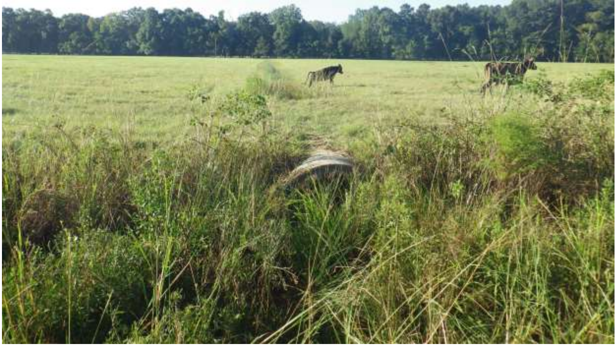
Culvert to be removed, Proposed Beaver Creek Mitigation Bank (photo taken September 27, 2017).
