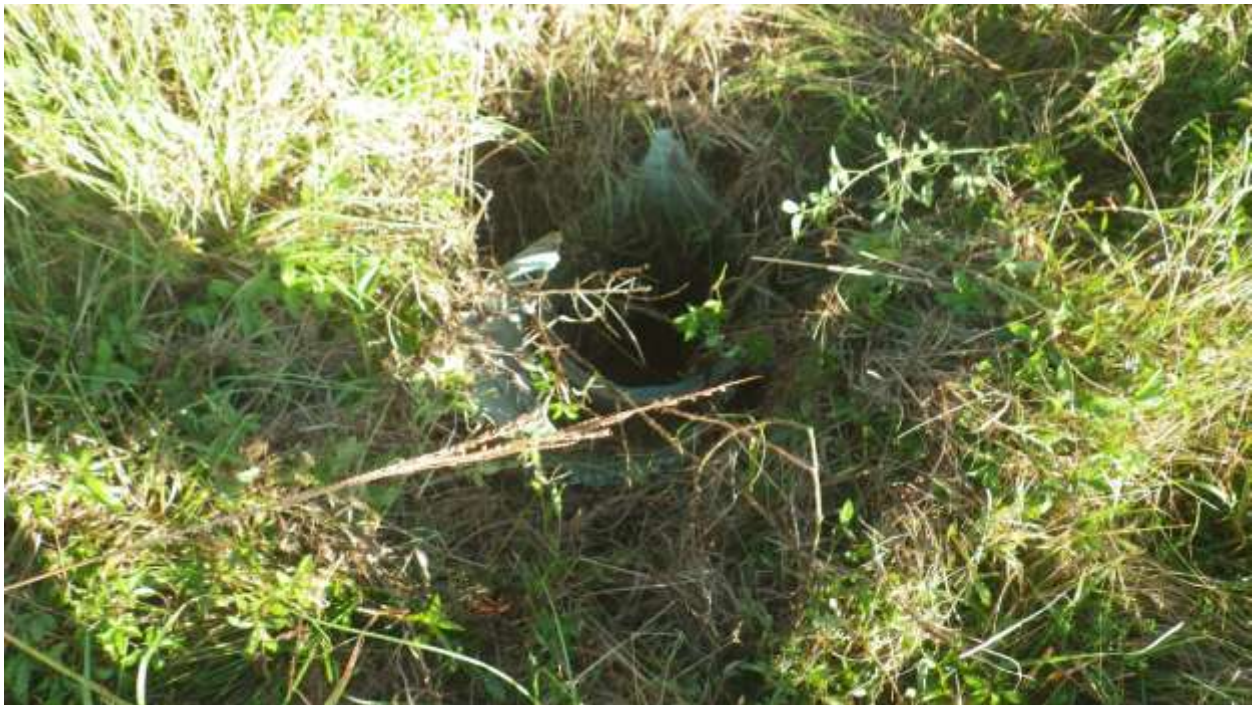
Subsurface drain to be plugged, Proposed Beaver Creek Mitigation Bank (photo taken September 27, 2017).
